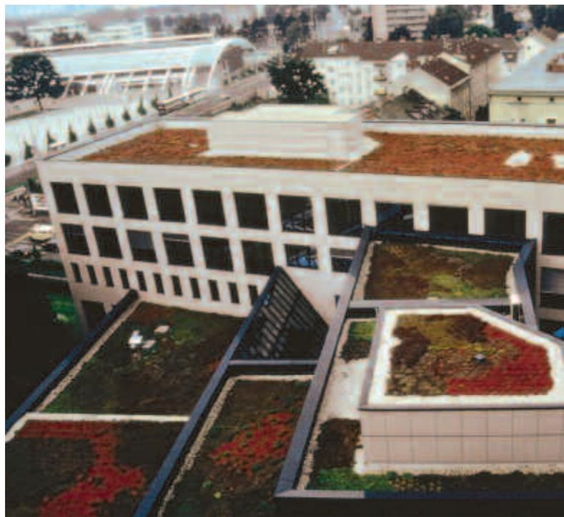
**In Germany, an entire service industry has formed around installing green roofs. Shown here is a two-inch-thick soil and vegetation roof cover used to control runoff (above) and a six-inch-thick cover (at right).**
